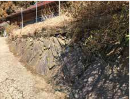
矢造変成岩の石積 Traditional stone masonry with regional ss(metamorphic rock)
